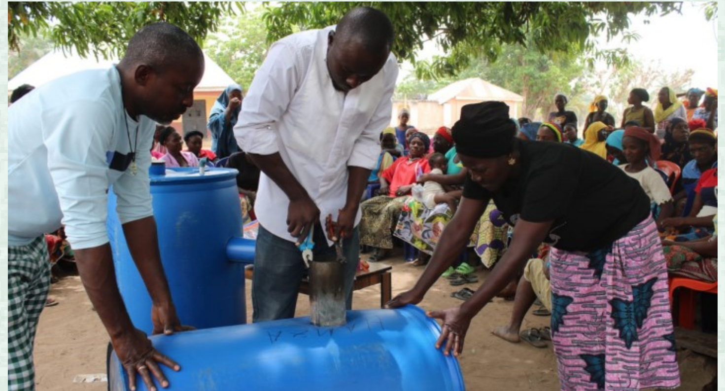
Demonstration of setup up of a bio-gas digester during a training session in a community
