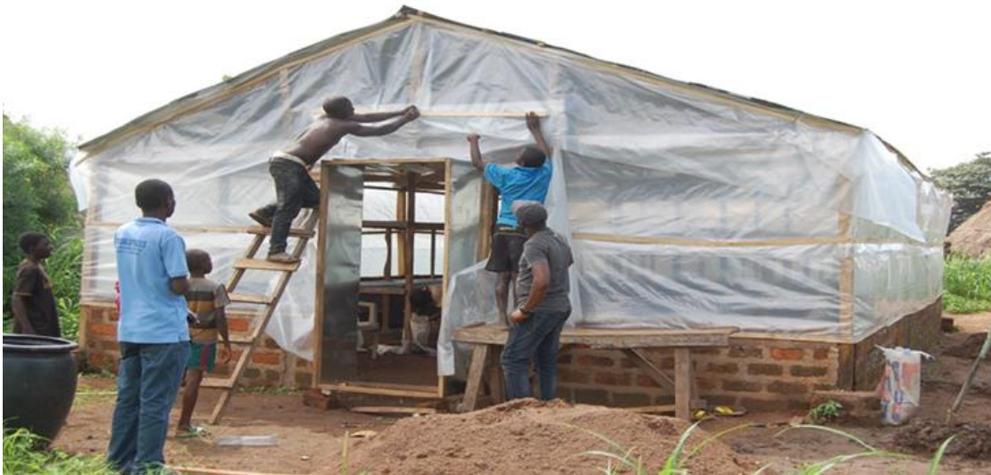
Solar dryer tent constructed in Adogo community
