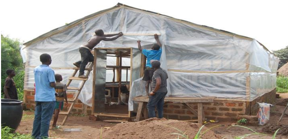
Solar dryer tent constructed in Adogo community
